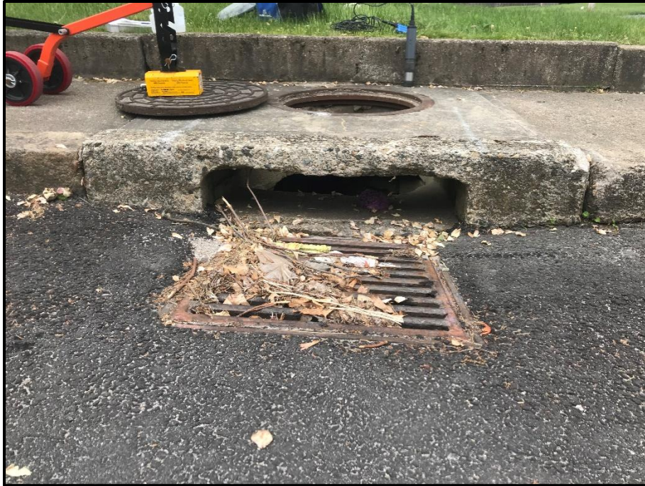
Photo 5: Manhole and catch basin on Lake Street.
