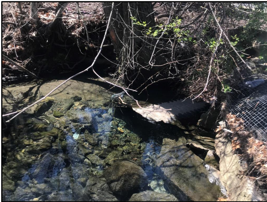
Photo 4: Stormwater outfall at the termination of Lake Street
