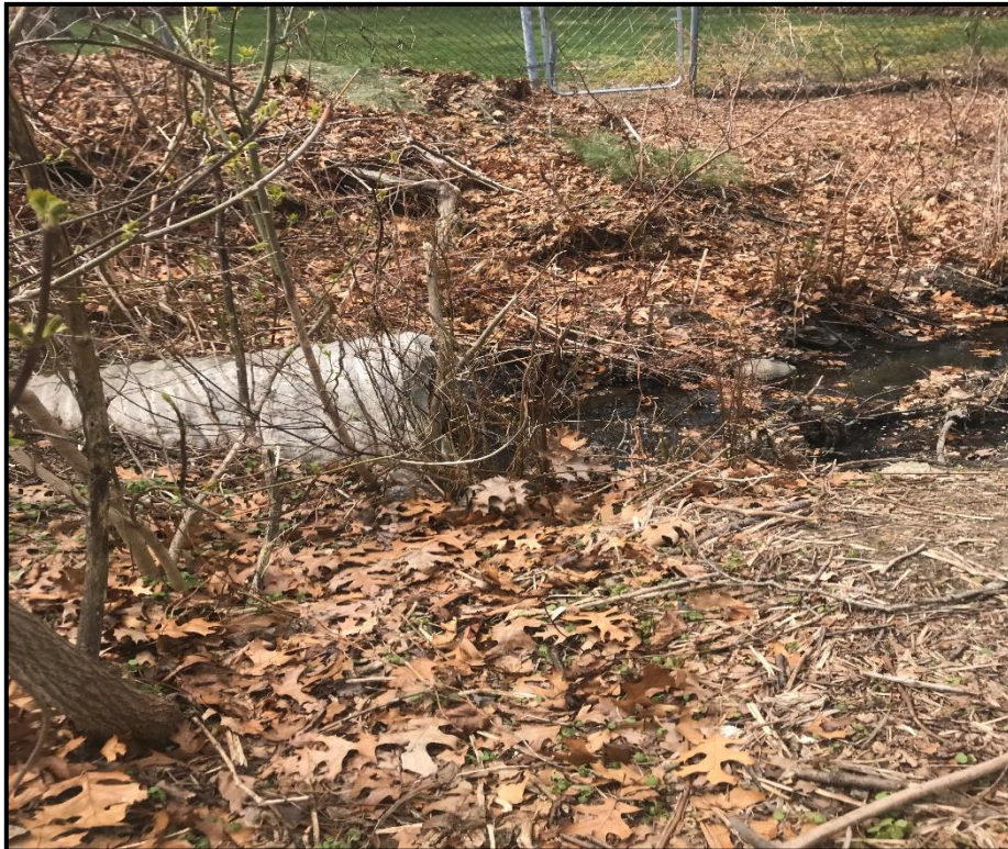
Photo 6: Stormwater outfall next to Speck Field
