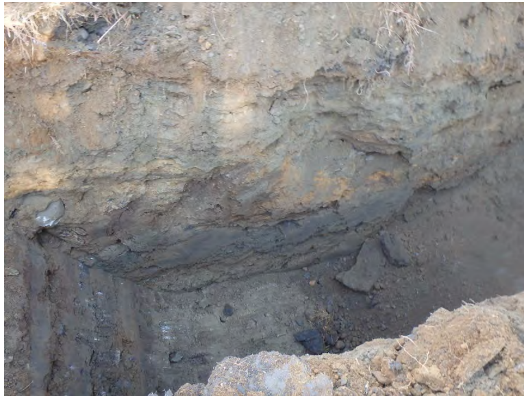
Photograph 4. Exposed fills to 2.6 meters (8.5 feet) below surface.
