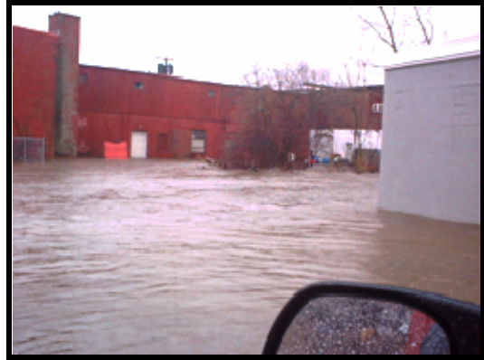
Photo 2 - Flooding at a Mill Complex on Simmons Brook west of Atwood Avenue, Town of Johnston
